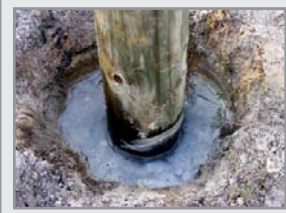
Water is present in the hole
