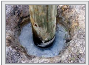
Water is present in the hole
