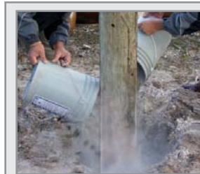
Pour in enough POLE QWIKSET as needed
